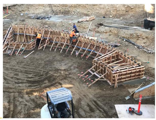
Amphitheater Retaining Wall # 2 concrete pouring
